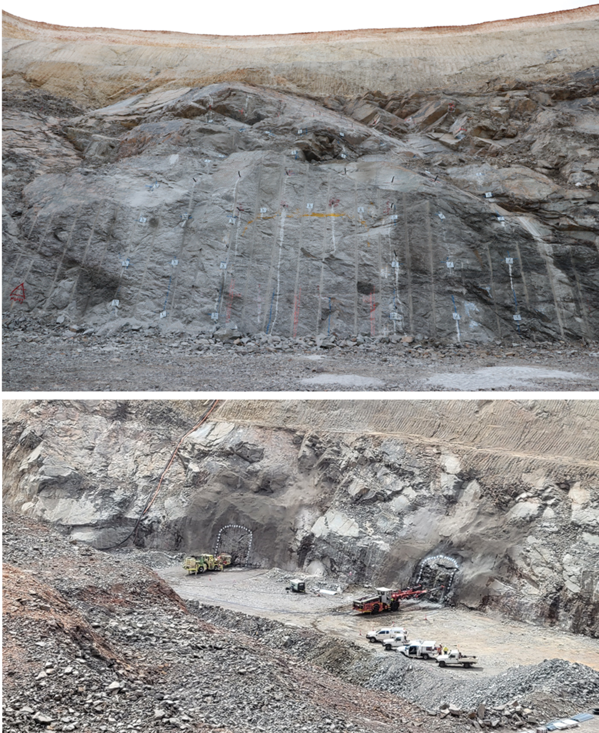
Figure 6 Completed ground support
